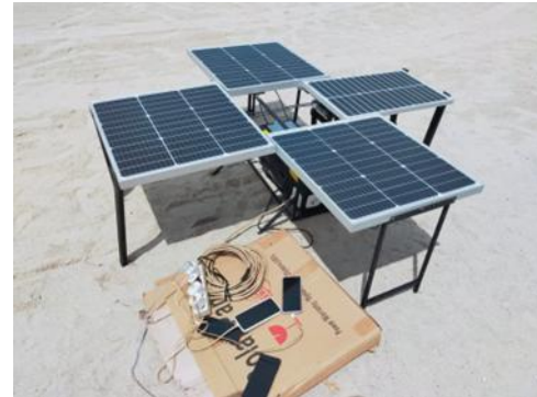
Figure 11. Charging a solar panel battery using a load.
