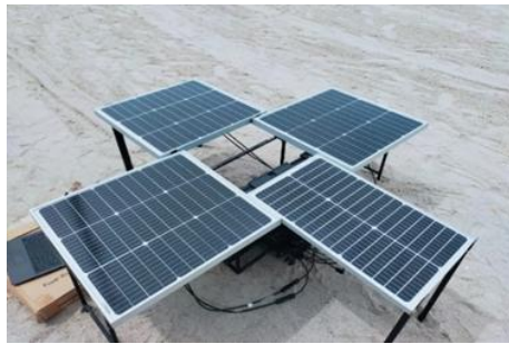
Figure 6. The results of the construction of the solar PV system.
