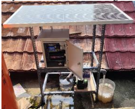
Figure 5. The results of the construction of solar PV.
