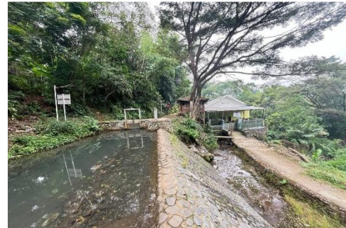
Figure 5. Photo on the Field.
