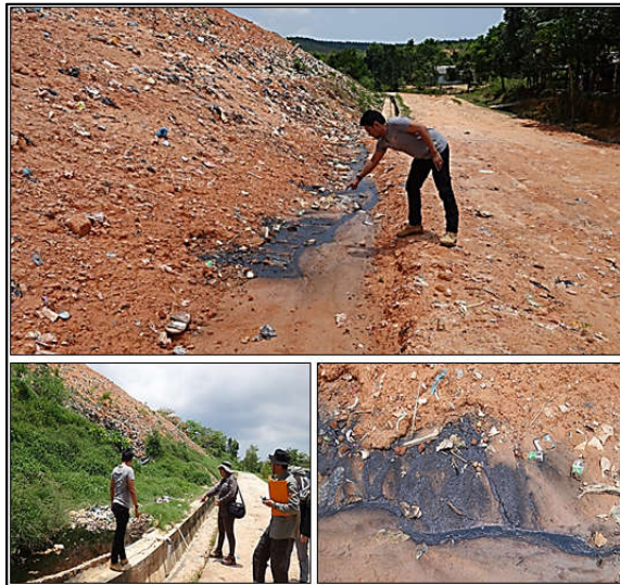
Fig 5. Black leachate in the Ganet waste processing site seeps out of control. Leachate is unable to penetrate the cover soil at the bottom of the waste landfill.
