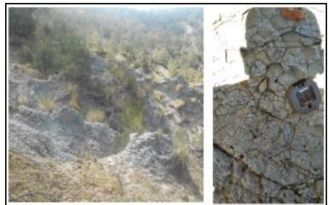
Fig. 6. Disintegration appearance and cracks on surface of Bobonaro Formation siltstone.
