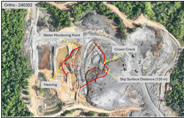
Fig 2. West Out Pit Dump Failure Scheme Elevation+30
