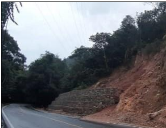
Fig 22. Landslide Mitigation with Retaining Rock Embankments
