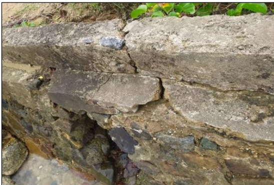
Fig 2. The Damage Condition Occurring on Almost the Entire Body of Tinobu Port's Causeway
