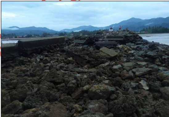
Fig 3. The Outer End Condition of Tinobu Port's Causeway Has Collapsed
