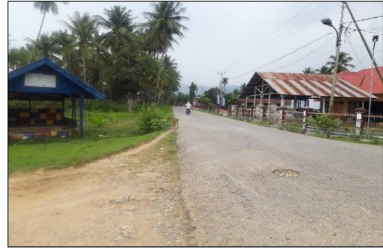
Fig 4. Condition of the Main Road in Front of the Harbor
