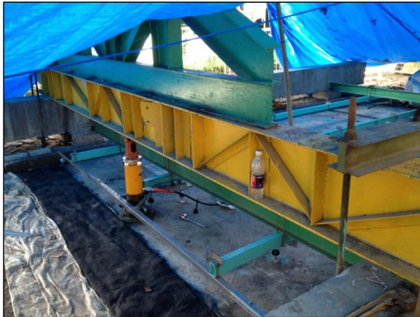
Fig. 2 Photographs of loading test on the edge of slab in the 3-pile row nailed-slab system (Puri, et.al. 2013b).
